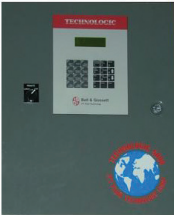
Bell & Gossett Technologic 5500 Pump Controller
